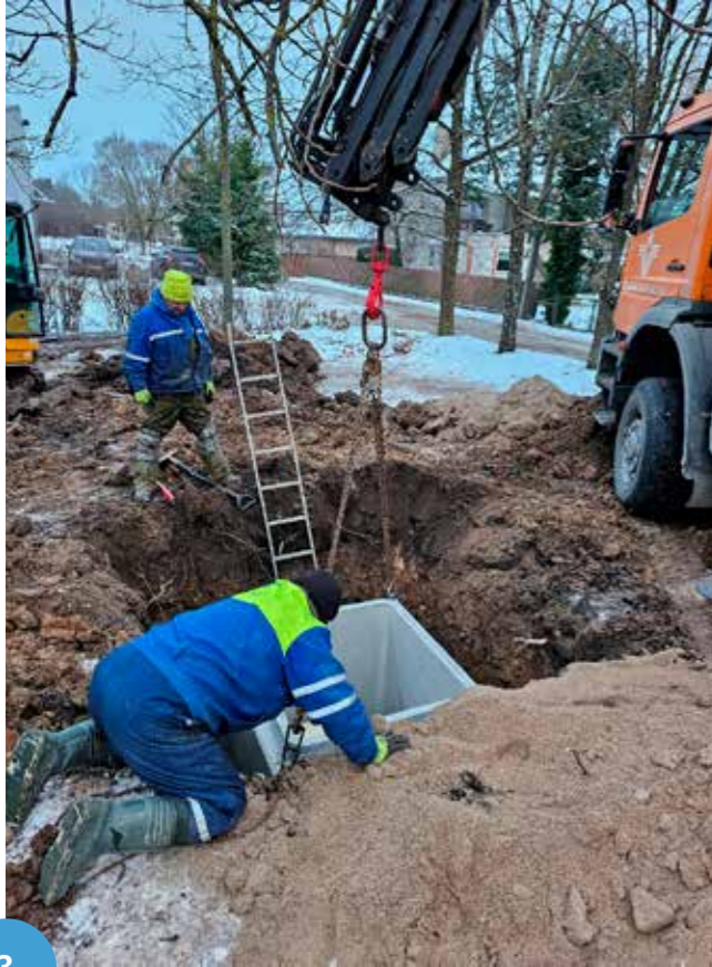
Preparation for the placing of the pre-treatment facility
