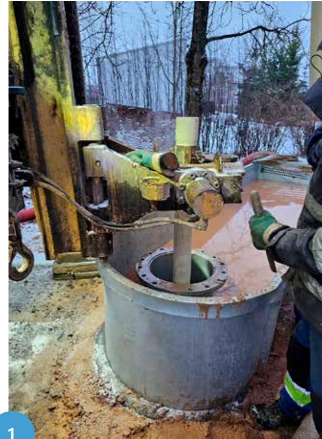
First drilling of the FHV well
